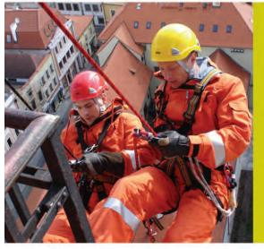
When using this rope, you will significantly increase your safety. Thanks to the unique sandwichtype construction of braided layers and the use of specially developed staple fibres, the rope is able to hold the suspended person or load even in case of considrably damaged sheath or core without the rope failing completely.
